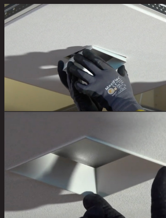
3 Insert USAI's Trimless Acoustical Trim
