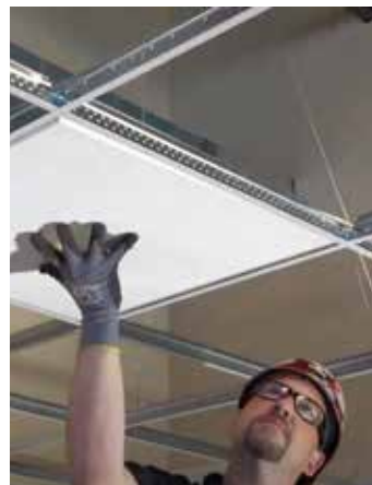
1 Place Precut Panel Into Grid 1" Cutting + Waste Eliminated
