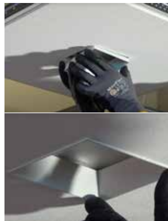
3 Insert USAI's Trimless Acoustical Trim
