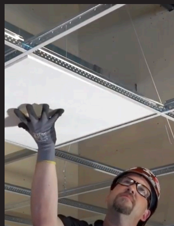
1 Place Precut Panel Into Grid 1 st Cutting + Waste Eliminated
