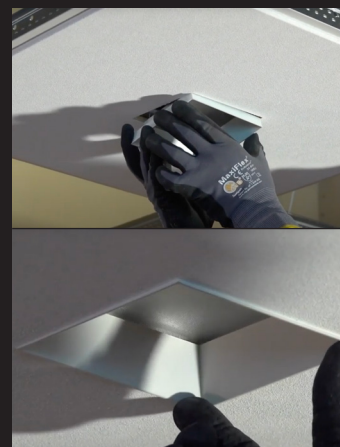
3 Insert USAI's Trimless Acoustical Trim
